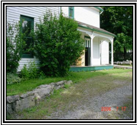
The back of the house before the addition of the rock and kitchen gardens
